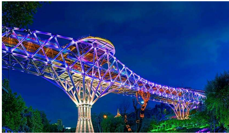
Fig.4 Tabiat (Nature) Bridge in Tehran – A user-centered, sustainable urban design project led by Iranian architect Leila Araghian.
